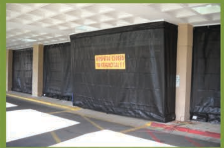
Large opening hurricane screens
